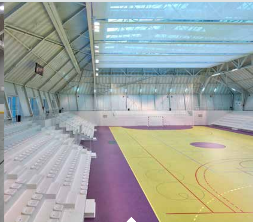
PALAIS DES SPORTS Loudeac, France Installed in 2014
